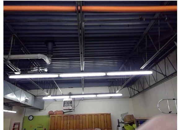
Attic / Roof Framing and Sheathing:
