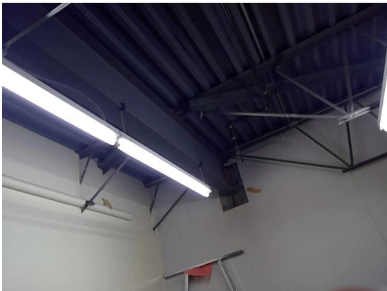
Attic / Roof Framing and Sheathing:
